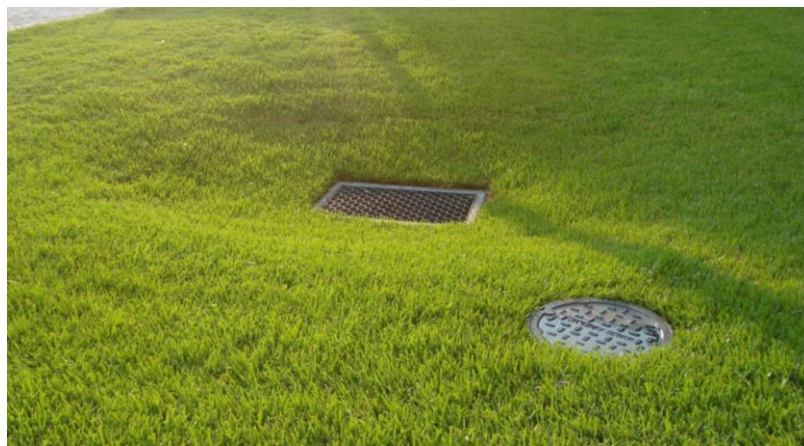
Figure 3.4.1.4 Park drain gutter
